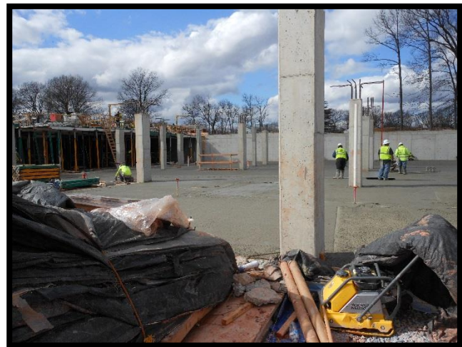
Figure 12. Structure of the Parking Garage
