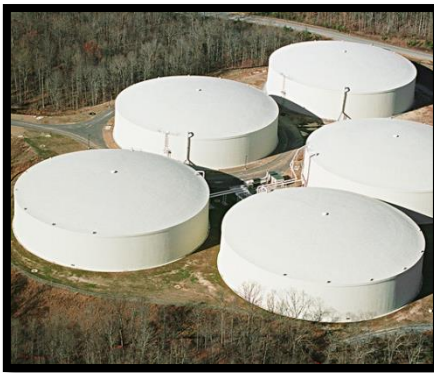
Figure 26. Prestressed Concrete Tank
