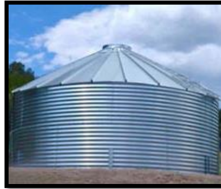
Figure 25. Above Ground Steel Tank
